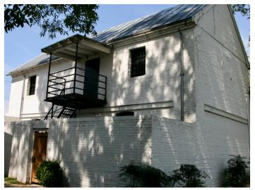
building sailing ships. He used plans drawn by John Hawk, 52 years earlier in 1773. Hawk is the unproven architect of the 1767 Courthouse. Ebenezer built this 36' X 21' brick jail in English Bond pattern, later stuccoed. The first-floor walls are 29" thick, second story's are 24" thick, and the end walls are 18" thick.
