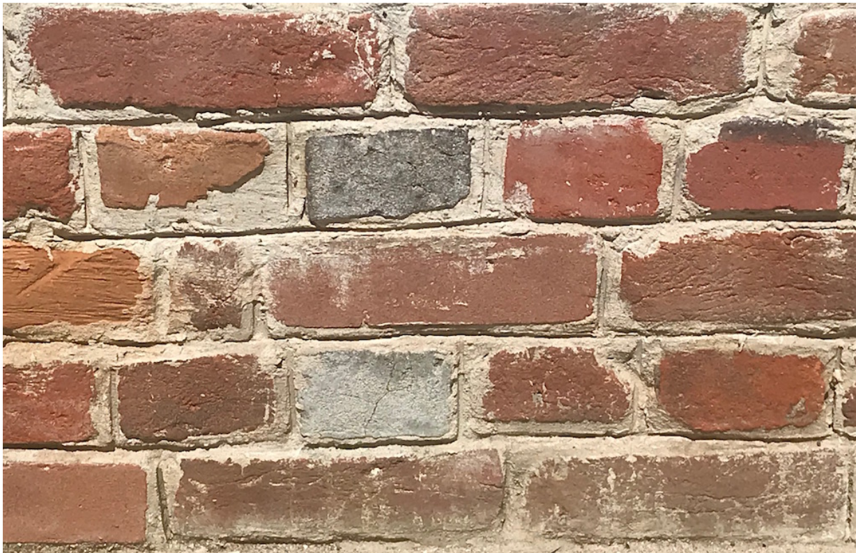
Figure 12, Cleaned brickwork
