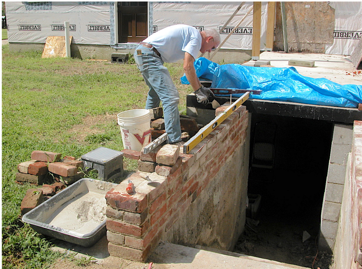
Figure 10, Brickwork base
