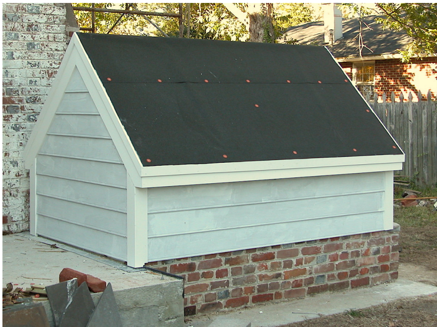
Figure 15, Siding and trim complete
