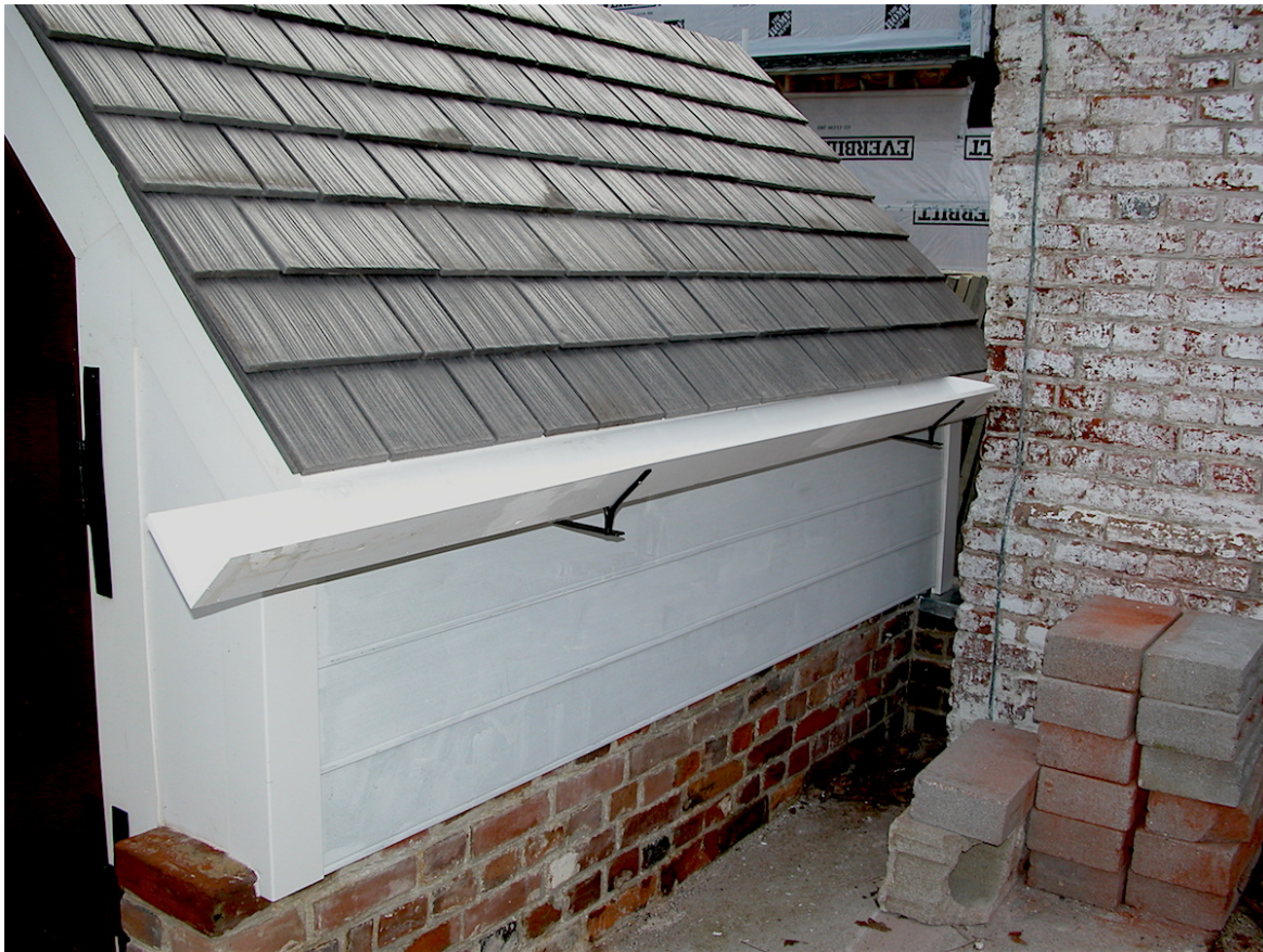
Figure 18, Roofing, eave gutter, and wrought-iron gutter brackets
