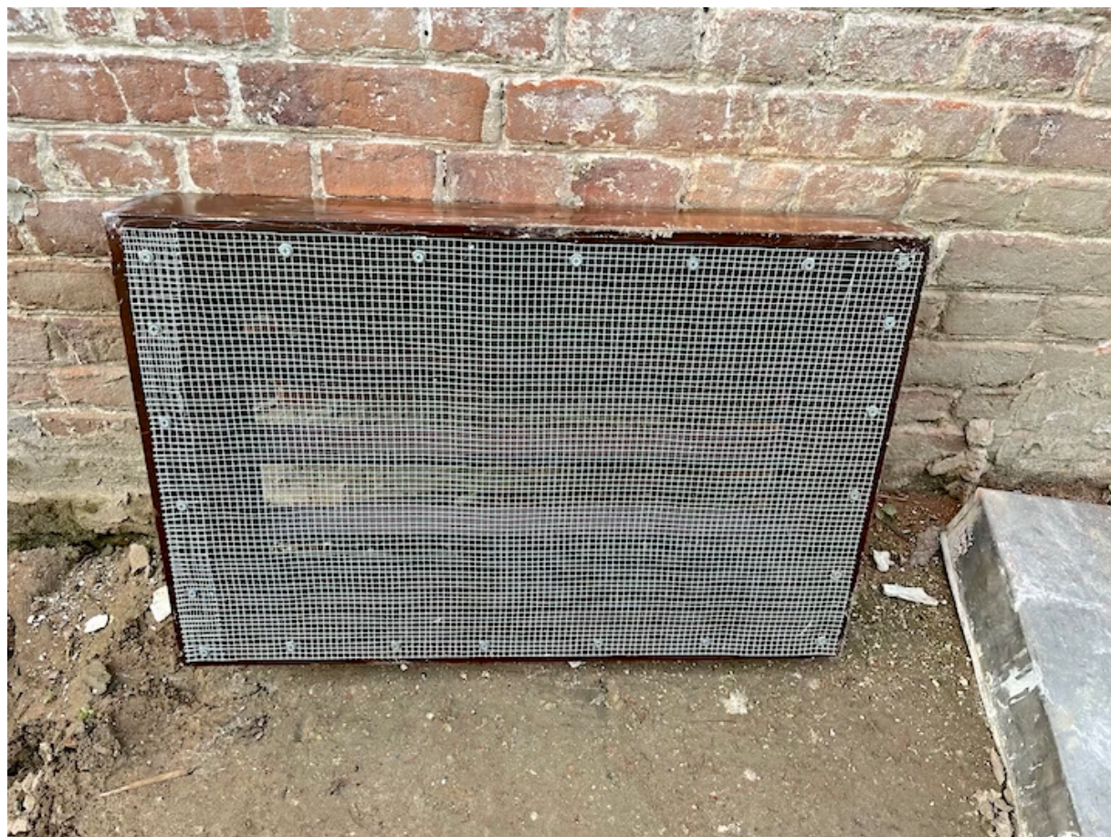
Figure 27 New vent with copper enclosed edges and rat wire.
