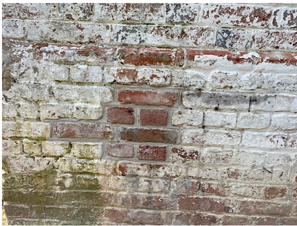
Figure 31 Joist pocket repair.
