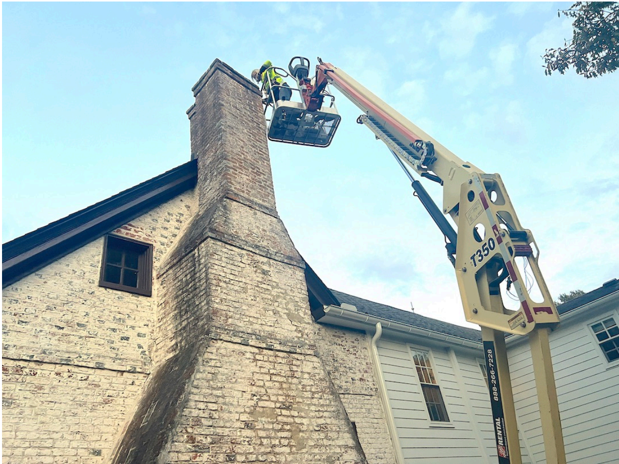
Figure 48 Chimney cap removal in progress.
