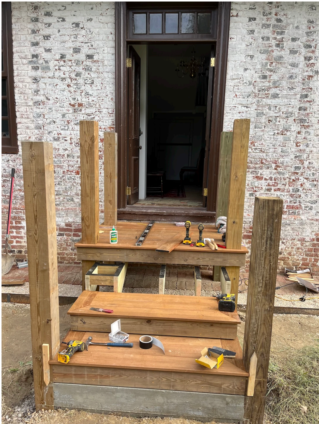
Figure 44 Entry steps and platform under construction.
