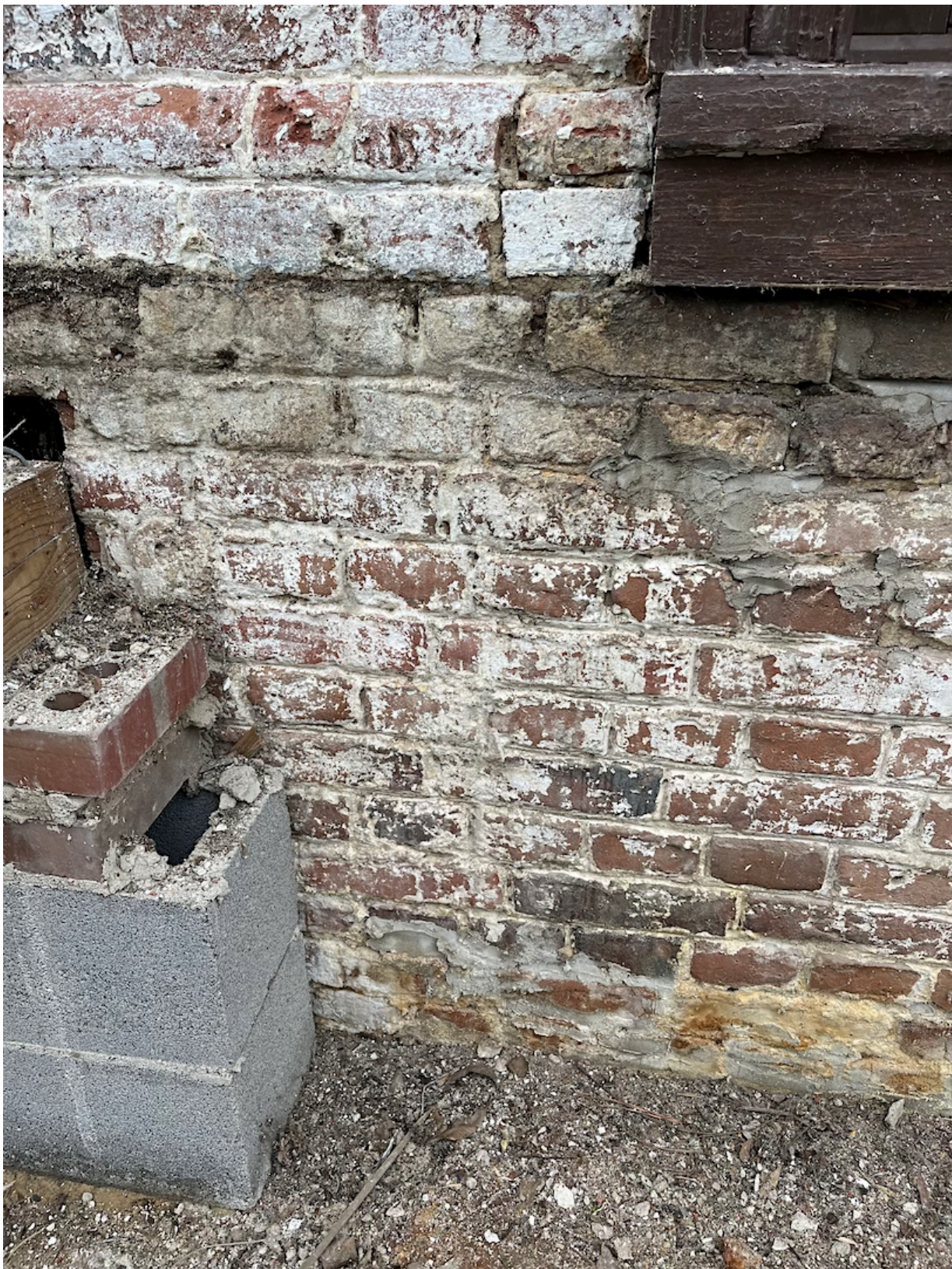
Figure 40 Clear vertical wear line to left of door below watertable.
