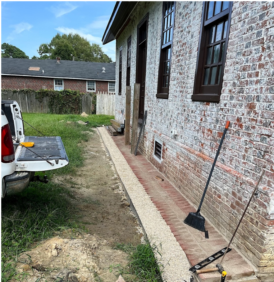
Figure 39 Finished ground gutter.
