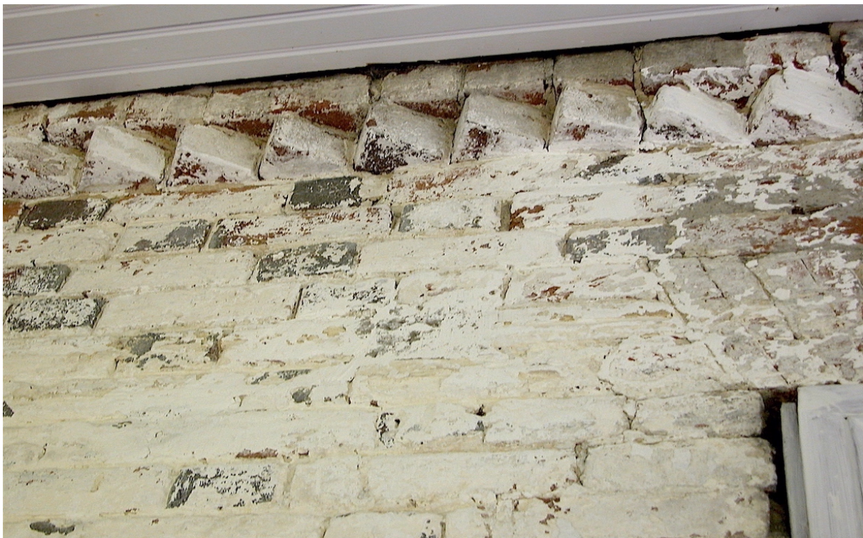
Figure 7 Detail of decorative toothed brickwork.
