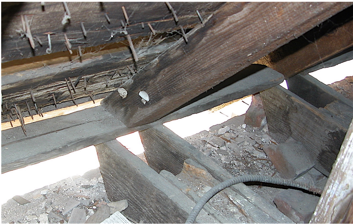
Figure 3 Circa 1815 roof structure that replaced tilt-plate eave.
