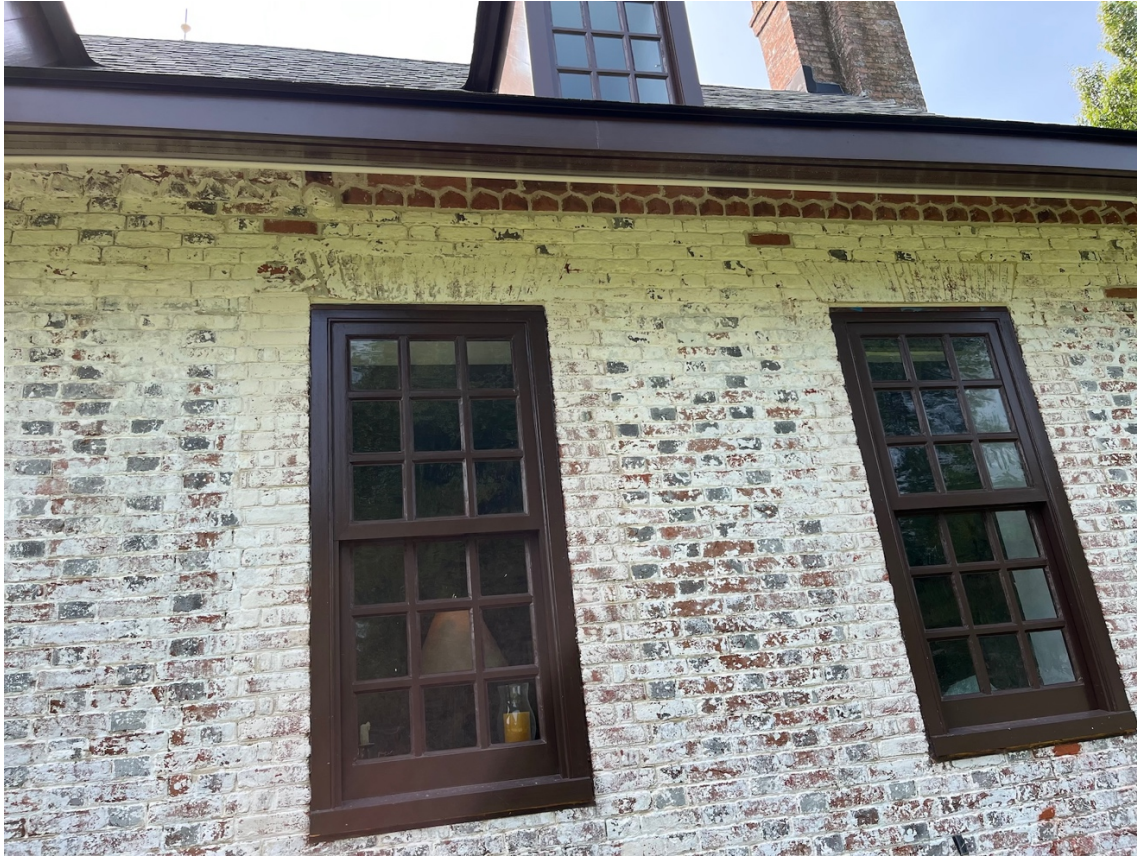
Figure 17 Both kick roof and brickwork complete.
