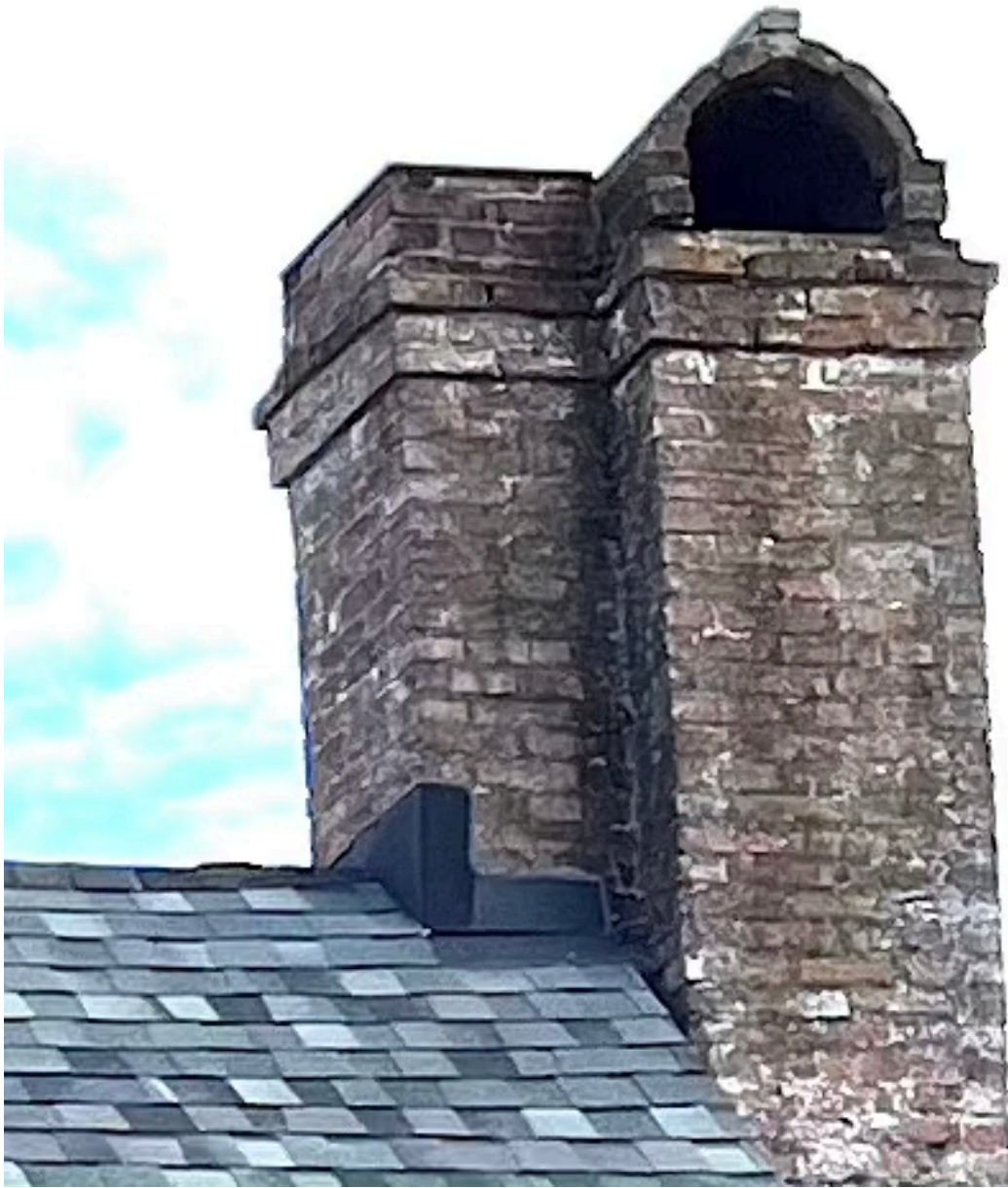
Figure 47 Chimney cap before removal.
