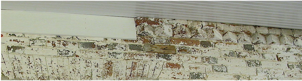
Figure 8 Fascia-type board covering areas of missing brick.
