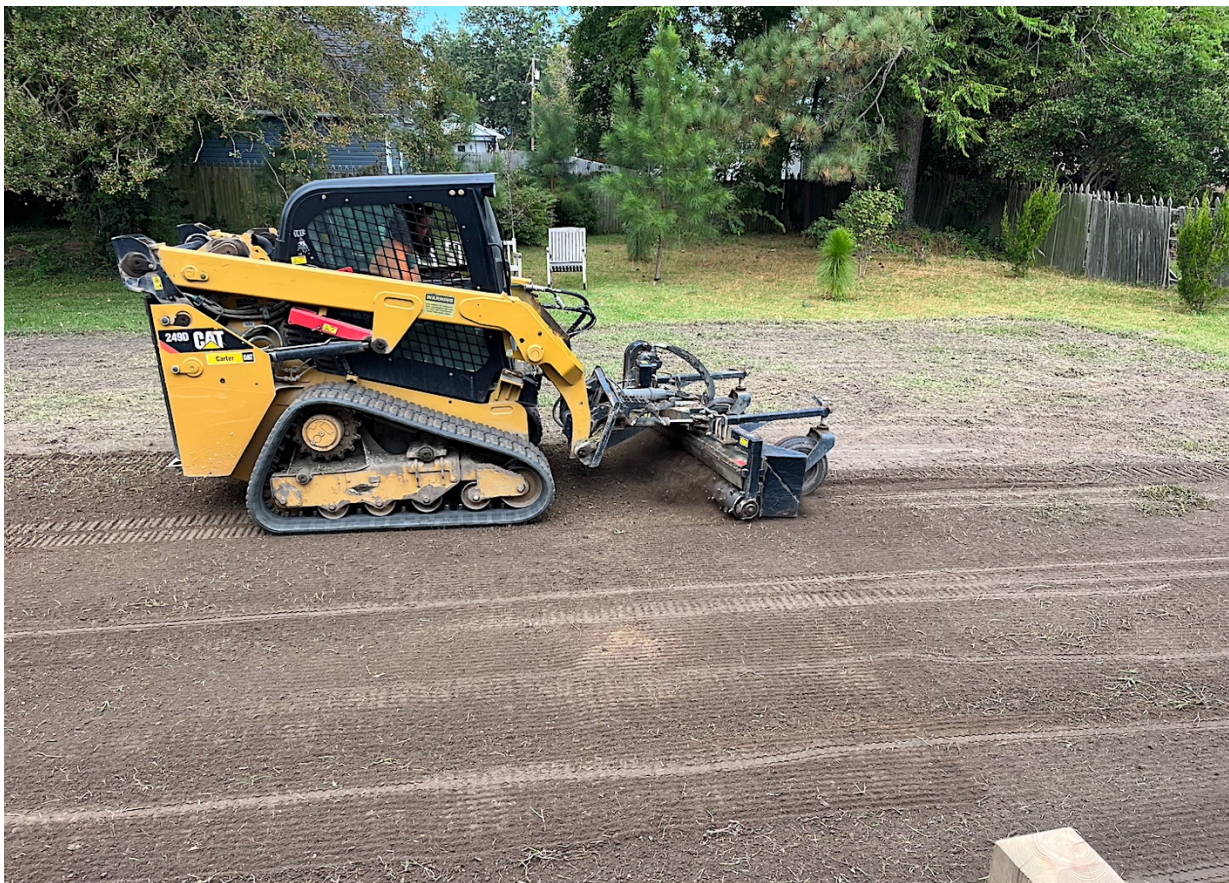
Figure 46 Grading for surface-water management.
