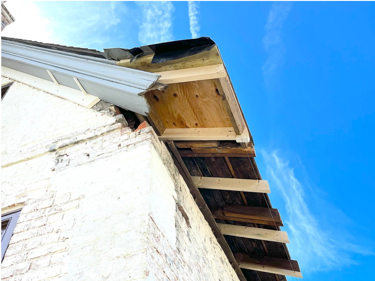
Figure 13 Framing for the kick roof and eave.
