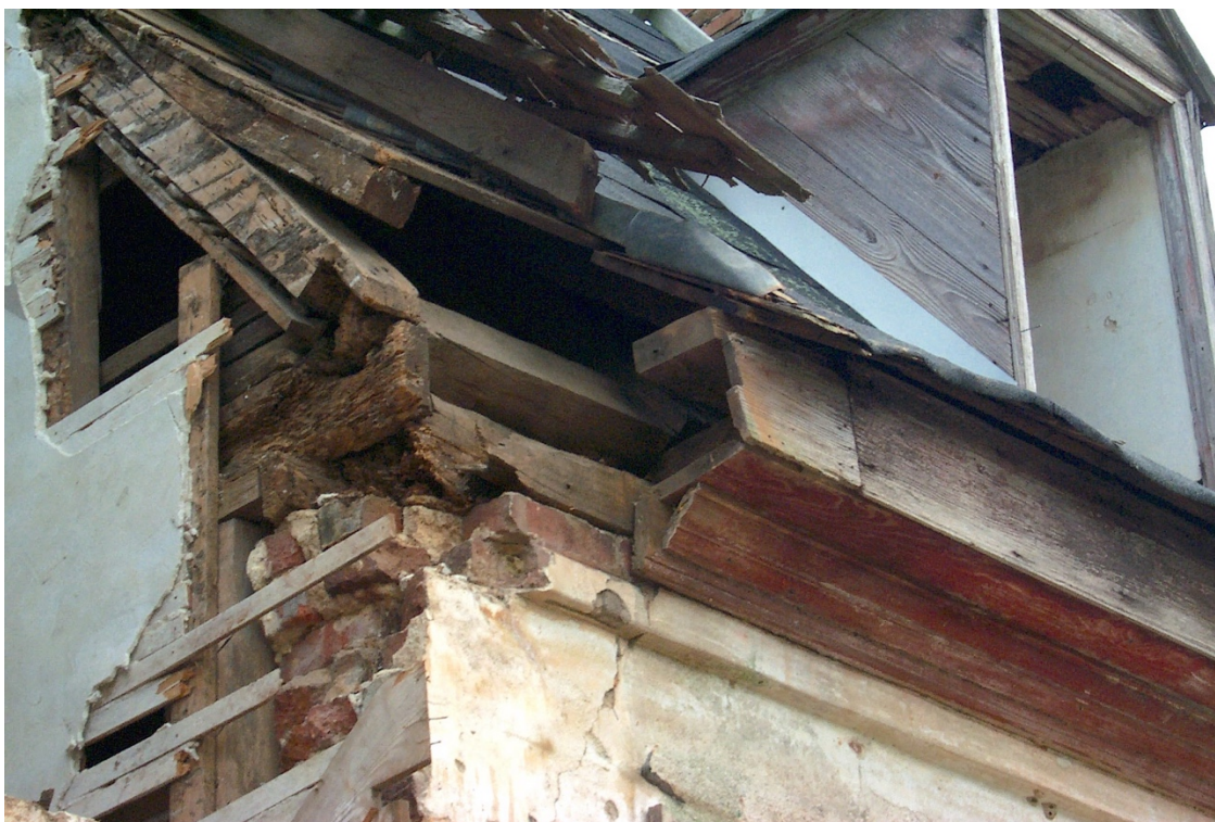
Figure 10 Original roofline kick construction detail on Mason House.
