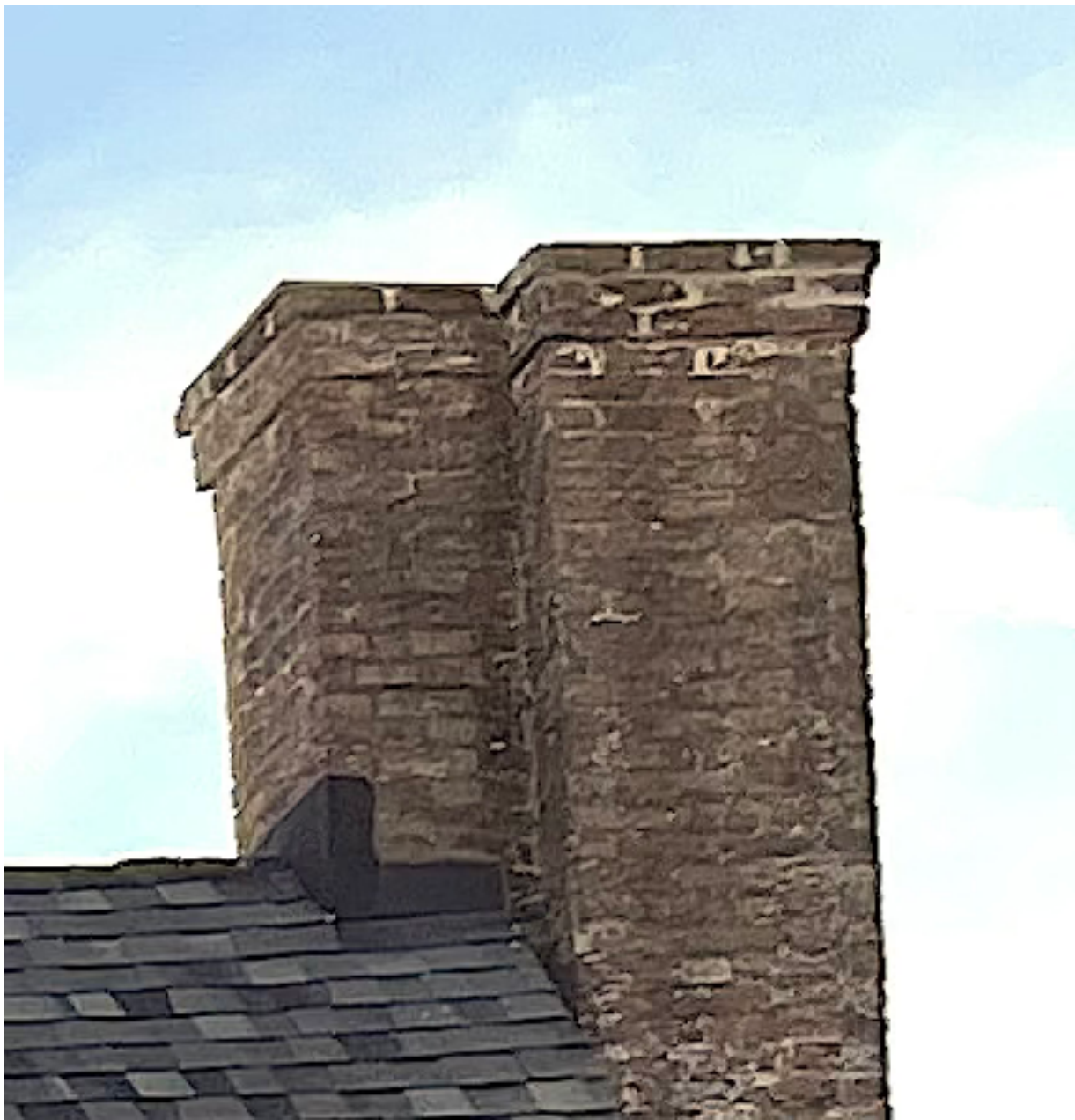
Figure 49 Chimney after chimney cap removal.
