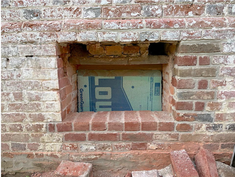
Figure 25 East opening ready for vent installation.
