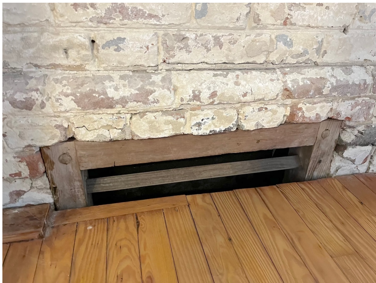
Figure 22 Original south barred vent.
