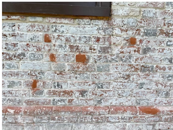
Figure 32 Brick repairs.
