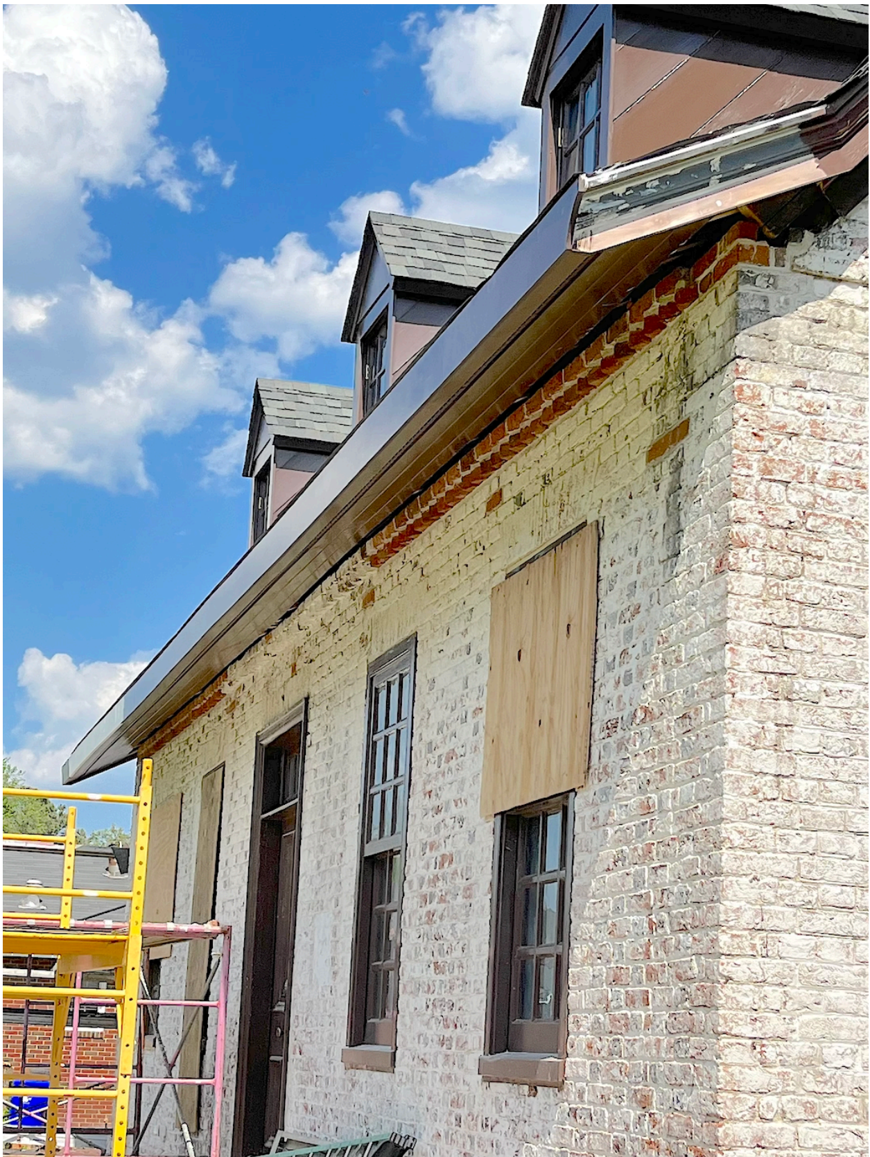
Figure 16 Brickwork complete, soffit of kick near completion.
