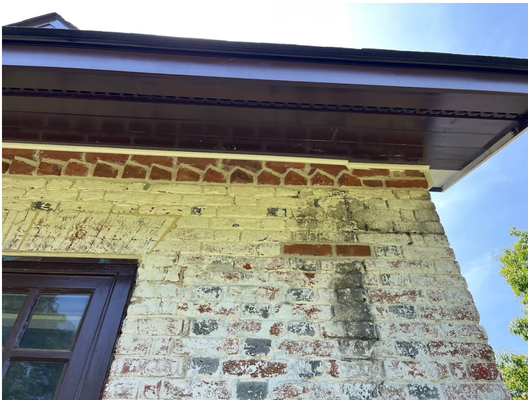
Figure 18 Area of missing corbel.
