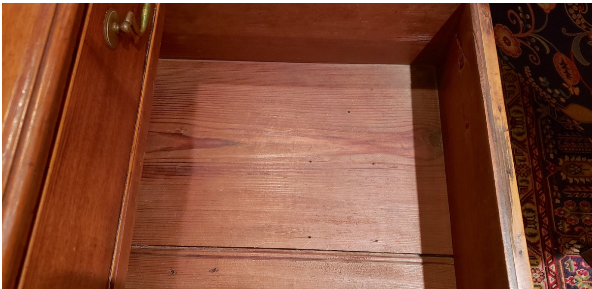
Figure 21 Beaded shiplap board used as drawer bottom in Fig. 20.
