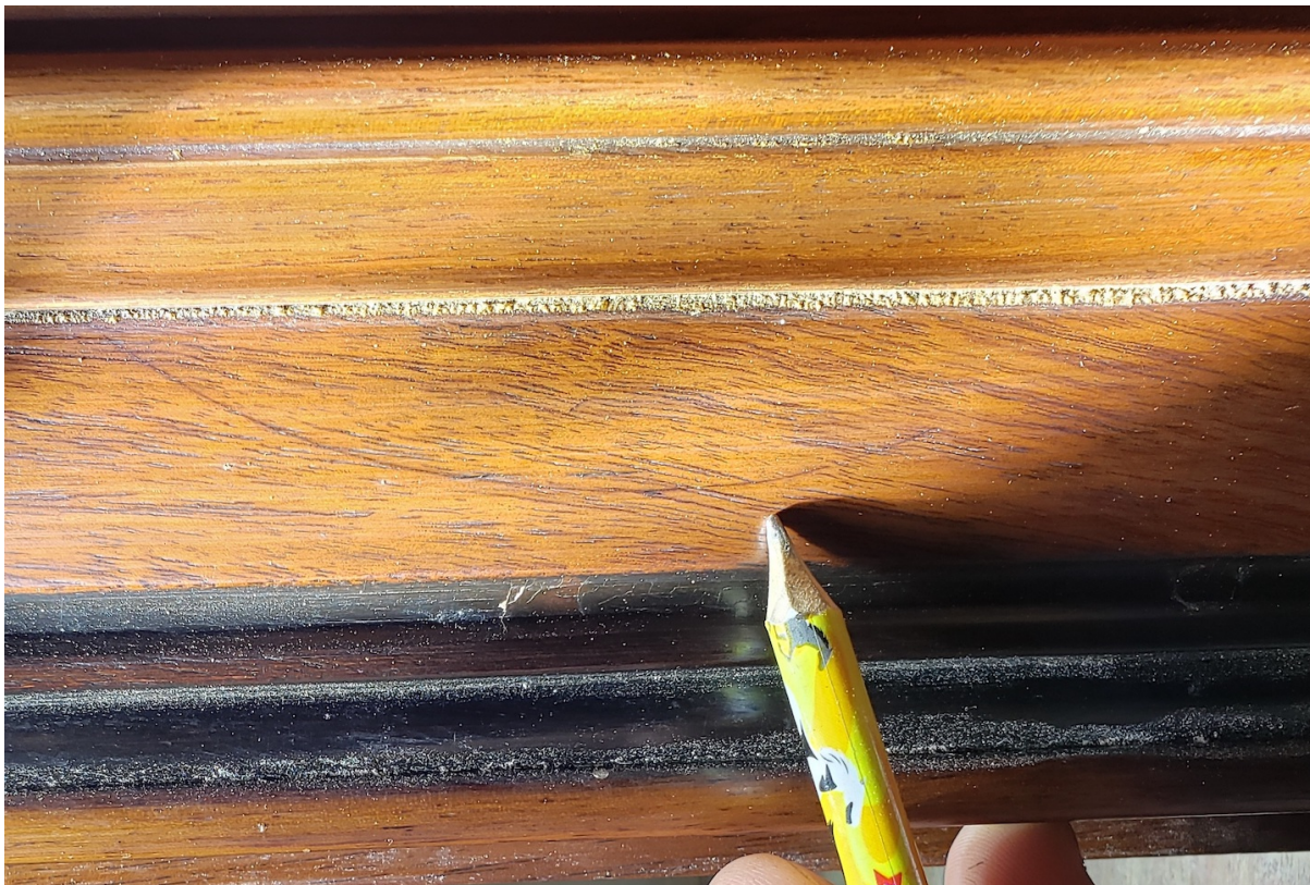
Figure 32 Marks on Fig. 22 consistent with letting-in relief carved leaves.
